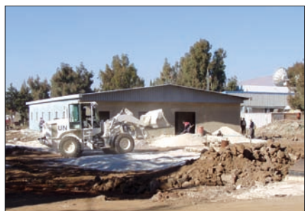
J-Con Heavy Equipment levelling the area around the new Medical Center
